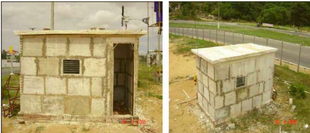
Figure 1 and 2: Houses built with Paines made from concrete with addition of EPS.
